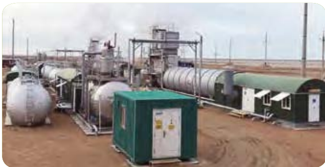
The four energy-saving boilers at Karazhanbas Oilfield
